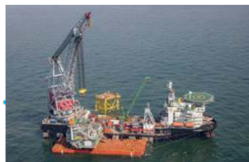
Galloper substation (UK)
